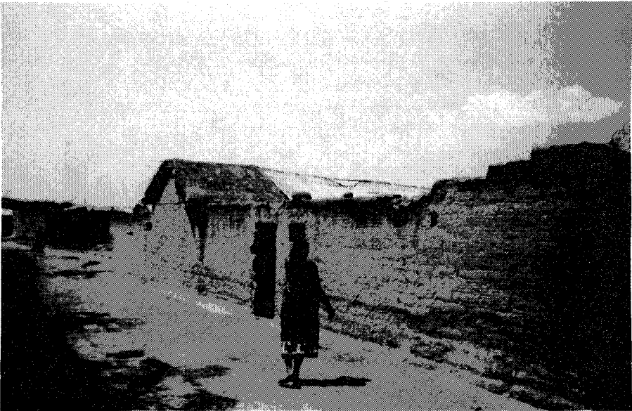
Fig. 4 Replacement of traditional building materials is a progressive process. Here, in Tanzania, thatch roofs are being replaced as corrugated iron sheets become available.
